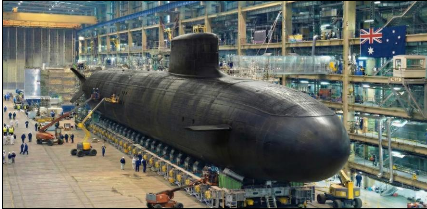
Outline plan for the yard at Osborne, which has three distinct areas.
