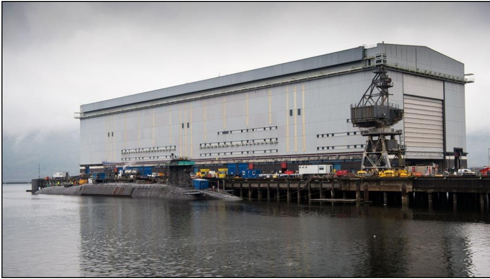
A Vanguard-class submarine undergoes maintenance at HM Naval Base Clyde at Faslane (Photo by ANDY BUCHANAN/AFP via Getty Images)
